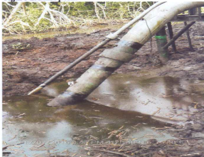
FIGURE: 3 REPAIR WORK
